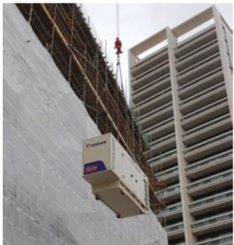
Teksan supplied, commissioned and installed a 230 kVA Diesel Generator in London, Kings Cross.
