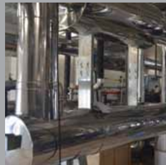
Exhaust Gas Heat Exchanger
